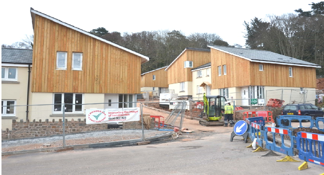
© ENPA Affordable Housing at Villes Lane Porlock under construction
