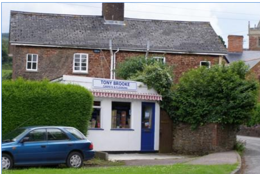
© ENPA (2009) – former shop at Timberscombe
