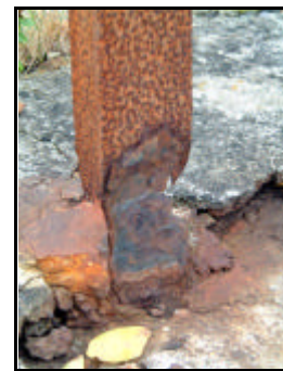
From left to right :: Poorly repaired surface at the Quayside. Deteriorating stable-block paving. Cobbles and edging stones in need of restoration. Evidence of severe sea erosion of metal railing.
