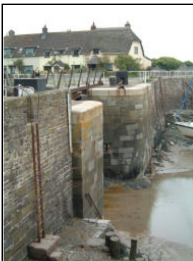
The present quayside is mainly 19th century, and not a weir so much as a tidal inlet which can be controlled by lock gates
