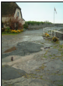
From left to right :: Poorly repaired surface at the Quayside. Deteriorating stable-block paving. Cobbles and edging stones in need of restoration. Evidence of severe sea erosion of metal railing.
