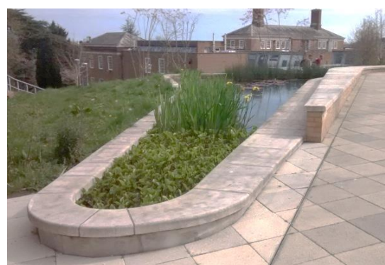
Figure 8: this well-planted attenuation pond serves the University of Exeter's Forum building by collecting, attenuating and treating the surface water runoff from the roof, whilst also providing a biodiversity and amenity benefit to the users of the area. Credit: Christopher Perrott (2016).
