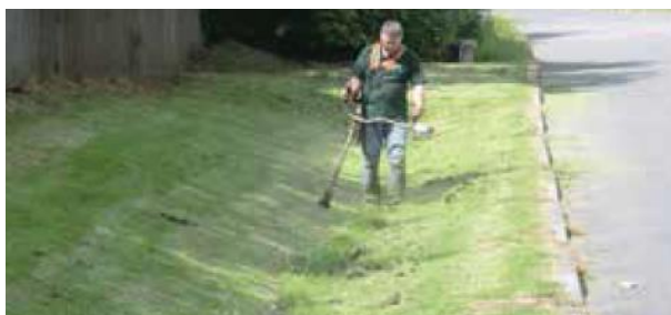
Figure 14: the maintenance of many SuDS components typically involves only a small amount of additional work (if any) over and above what is necessary for standard public open space. Credit: CIRIA C753 (2015), p. 328.
