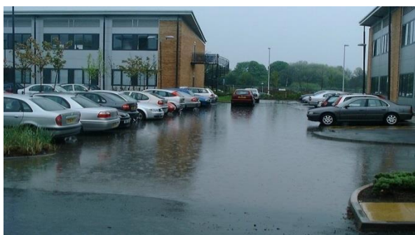
Figure 12: temporary ponding in car parks can manage surface water during extreme rainfall events, without placing the critical site infrastructure at risk. Credit: Susdrain (2016).
