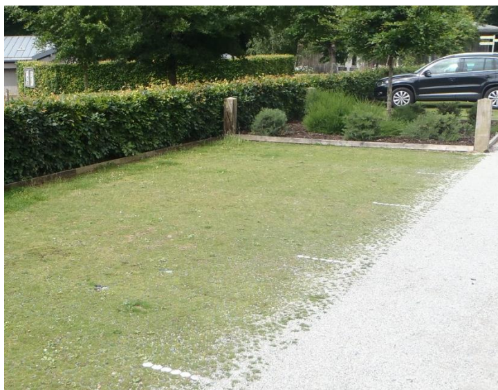
Figure 10: rather than attenuating the surface water runoff generated from this car park in Devon, a reinforced permeable surface has been used to allow infiltration into the ground. This method not only manages water quantity and quality, but also supports soil moisture levels and promotes vegetation growth. Credit: Christopher Perrott (2016).
