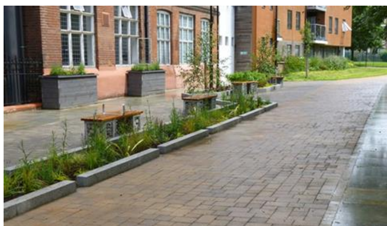
Figure 6: this linear rain garden receives surface water runoff from the adjacent footpaths, and is only approximately one metre wide; the land take and cost of such SuDS components can be minimal. Credit: Susdrain (2016).
