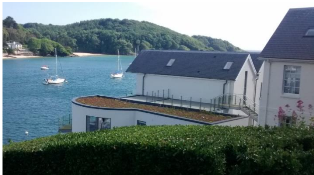
Figure 9: this green roof on a building in Salcombe manages the quality of the surface water runoff from the site before it is discharged, without attenuation, directly into Salcombe Harbour. Credit: Christopher Perrott (2016).
