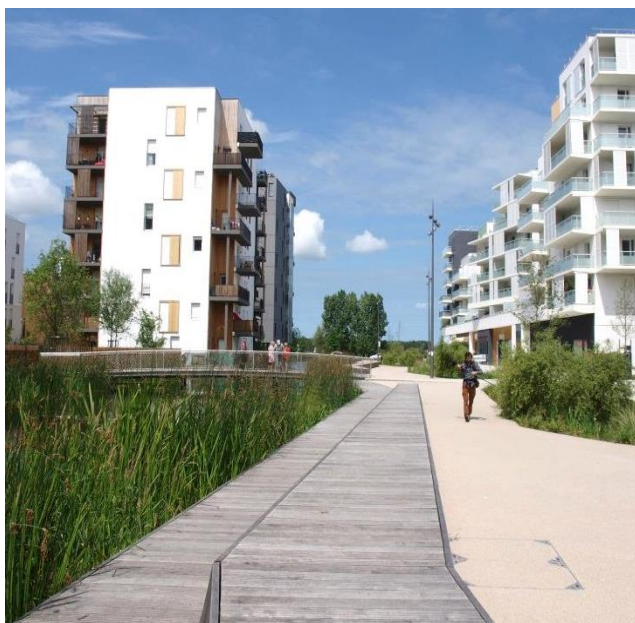
Figure 7: the surface water drainage management system for this development in Bordeaux was designed by a team of drainage engineers, landscape architects, ecologists and planners. This approach produced an effective surface water drainage management system which also enhanced biodiversity and ecosystem services, whilst aiming to improve public health and well-being. Credit: Sarah Foqué (2014).
