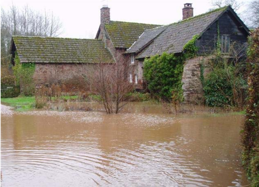
ENPA: house surrounded by flood water
