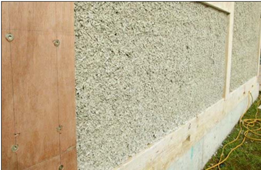
Figure 5. A hemcrete wall under construction.
