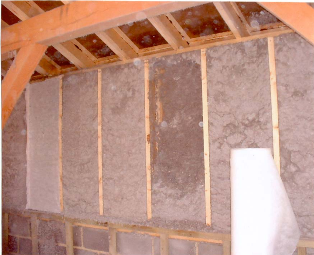
Figure 7. Wall detail showing insulation made from recycled newspaper.
