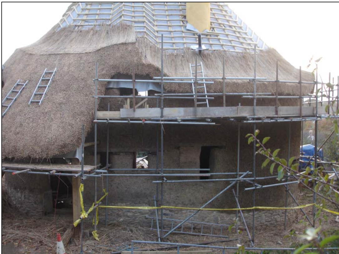
Figure 2. A new build cob house under construction in Devon
