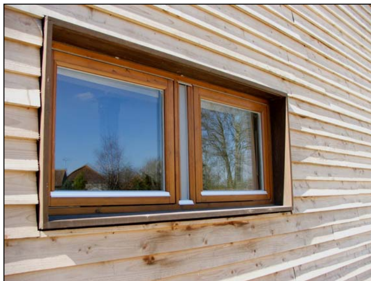
Figure 11. Sustainably sourced timber used as an external cladding.
