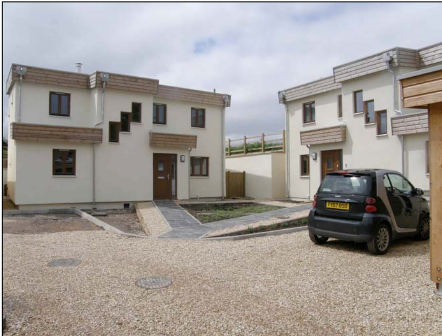
Figure 6. New build homes in Somerset rendered using lime.
