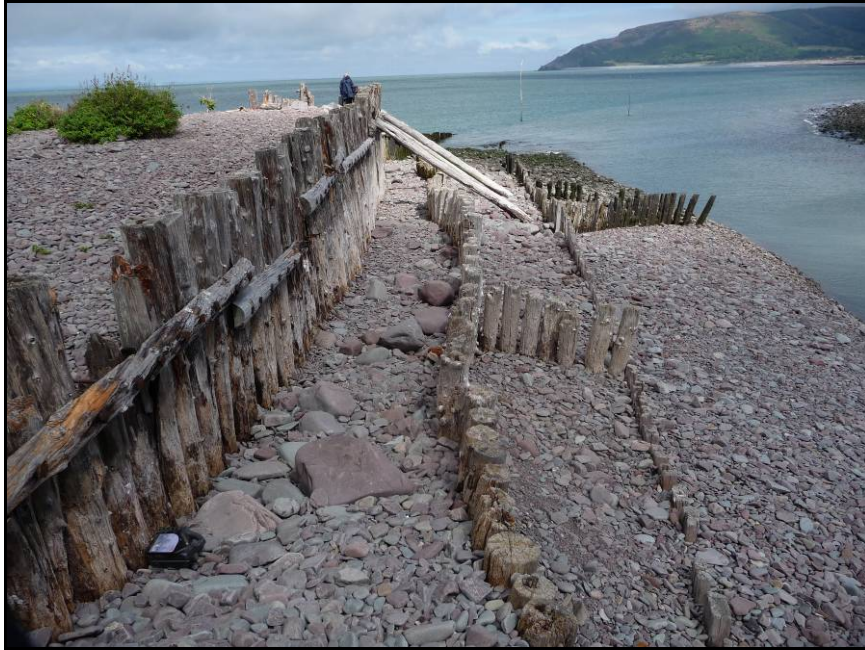
Figure 3.1. Timber groyne protecting the harbour at Porlock Weir
