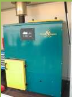
15-25kW pellet boiler
