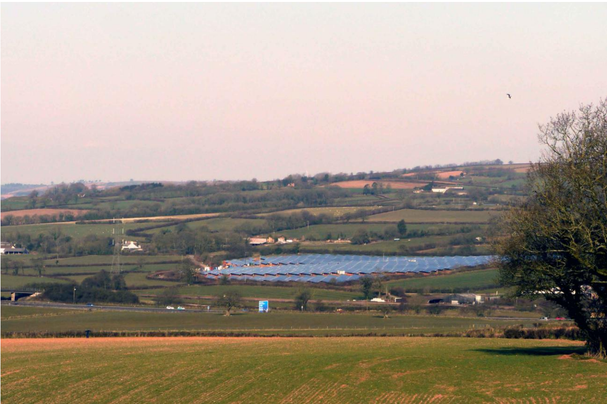
Solar PV Development at Ayshford Court Farm, Mid Devon (15Ha, upper end of the 'large' size category), photo credit: Andy Leithgoe
