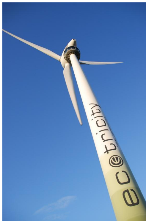
Example of graduated colours and company name on a turbine tower
