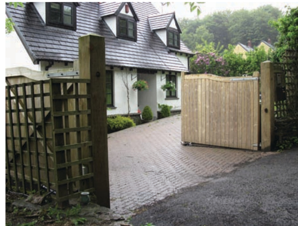
Recent development that weakens character, largely through the suburban character and management of the curtilage. Keeping curtilages to a minimum and out of public view, behind buildings and stonewalls, would help to conserve character
