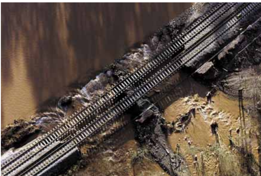
← The railway embankment at Cowley Bridge near Exeter was washed away by the River Exe just after it had been repaired following an earlier flood
