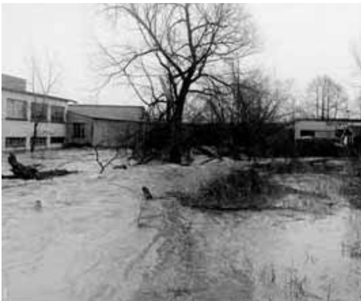
↑ Flooding of the Leather dressing works, Alexandria Industrial Estate, Cullompton - January 1984
