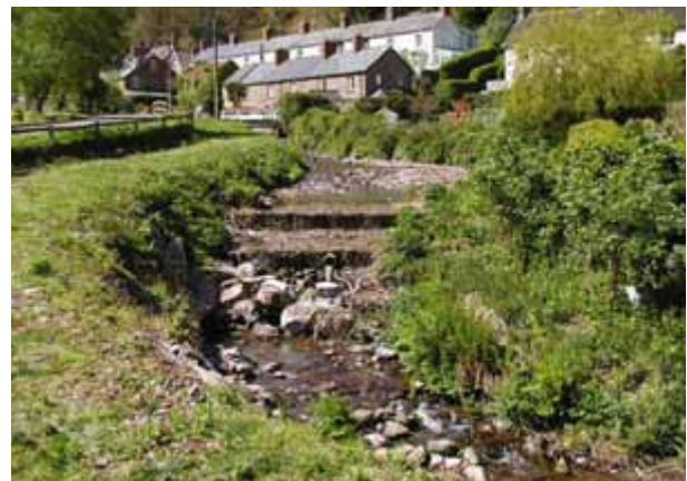
↑ A shingle trap on the Hawkcombe Stream at Hawkcombe
