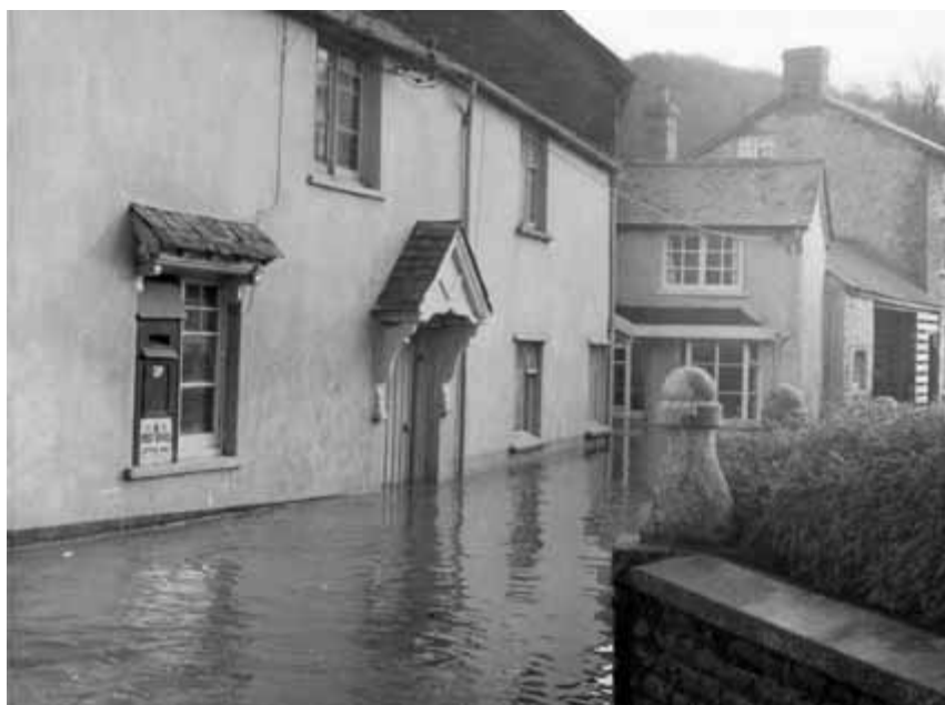
↑ Flooding from the Washford River at Roadwater in December 1965
