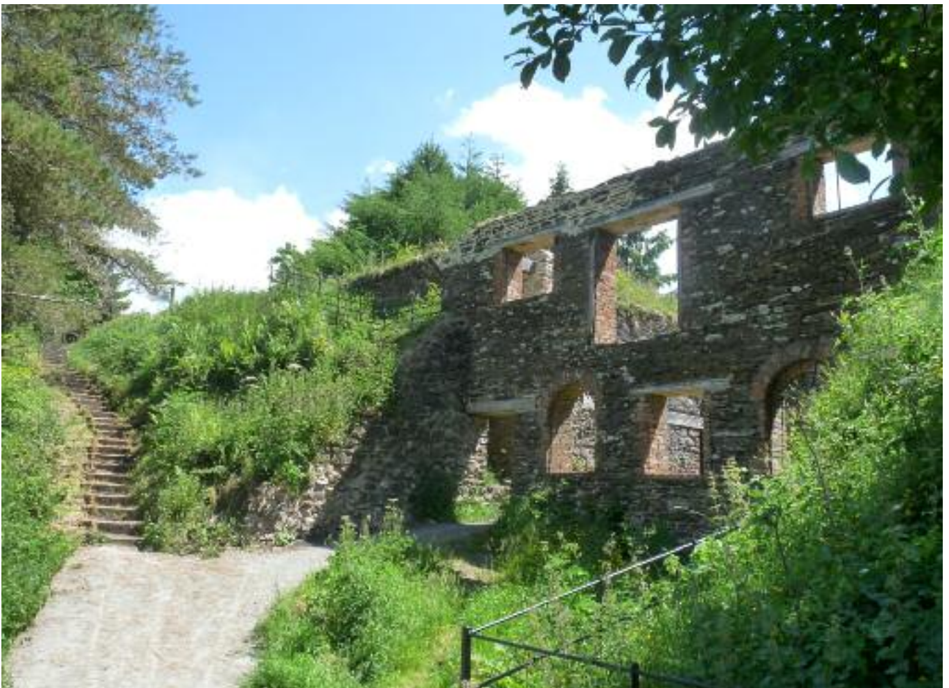
Ruined winding house at the top of the WSMR incline, Brendon Hill (constructed 1859)
