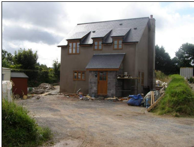
© ENPA - Intermediate affordable dwelling under construction
