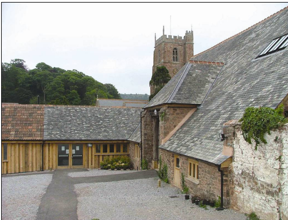
© ENPA: A stakeholder event was held at Dunster Tithe Barn in December 2008
