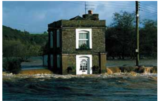
↑ A house at Taddiport marooned by the River Taw in October 2000 Photo: Clare Kendall
