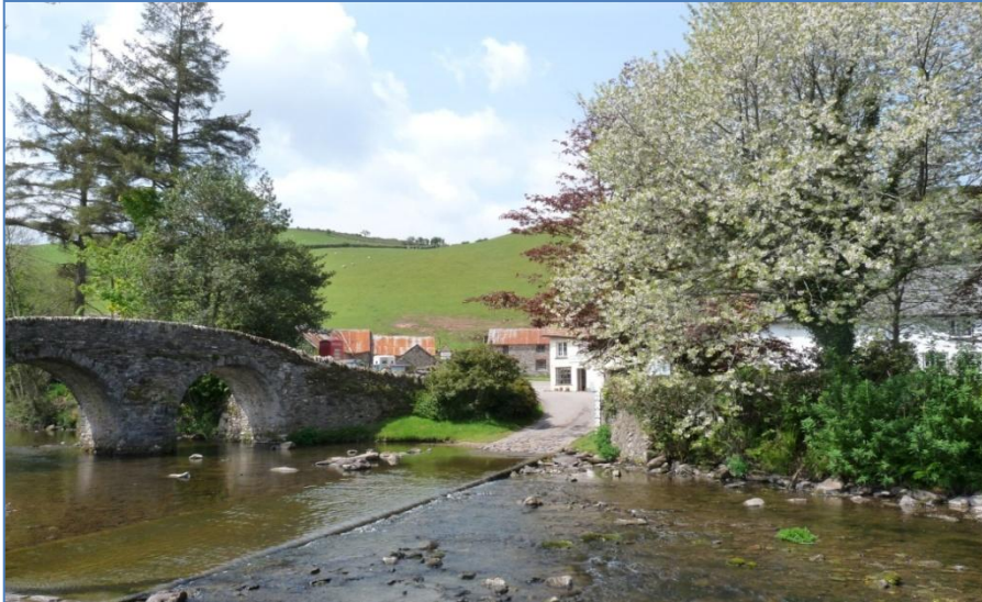
Malmsmead Bridge and Ford with Lorna Doone Farm in the background
