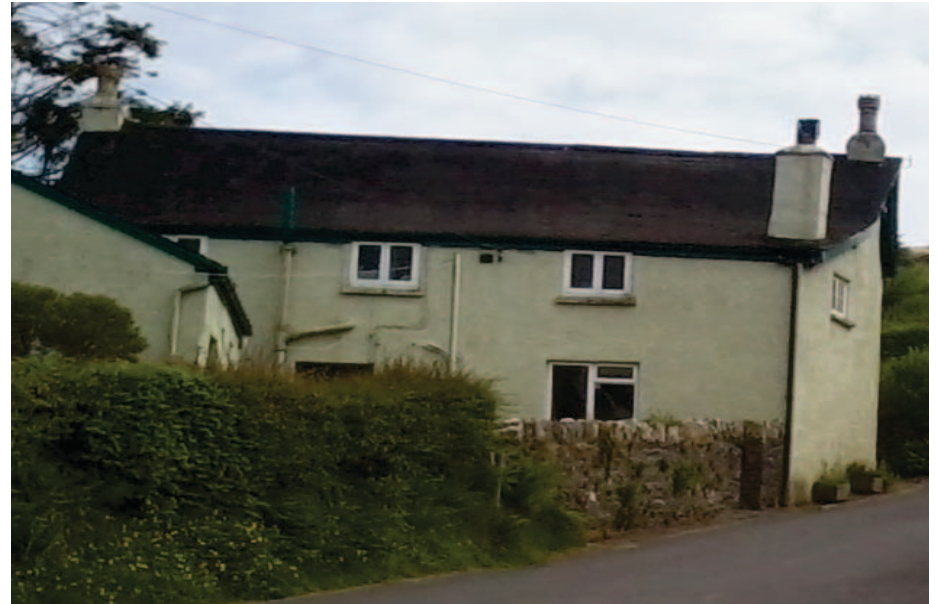
Vernacular small-scale cottage, rendered, with slate roof, abutting the highway with strong boundary and sitting in the landscape.
