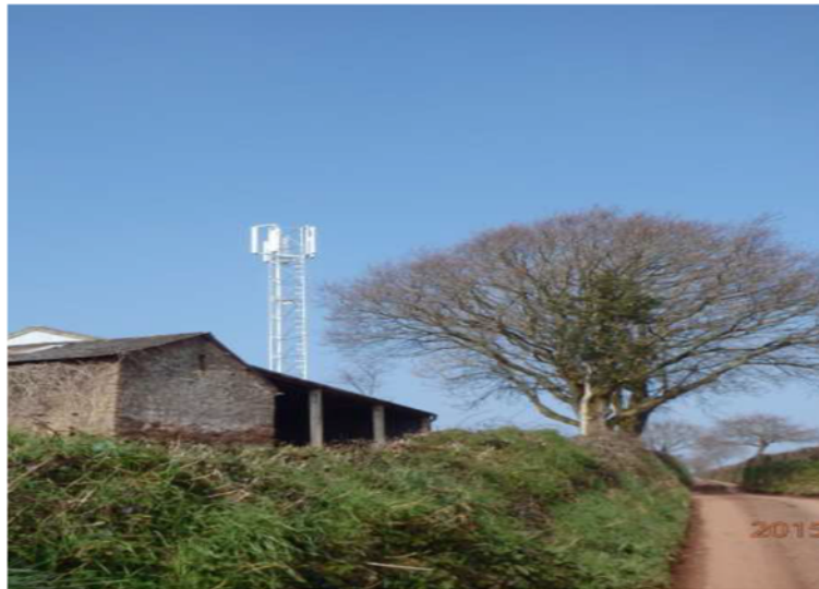
Shared telecommunications mast at Golsoncott Farm, Roadwater
