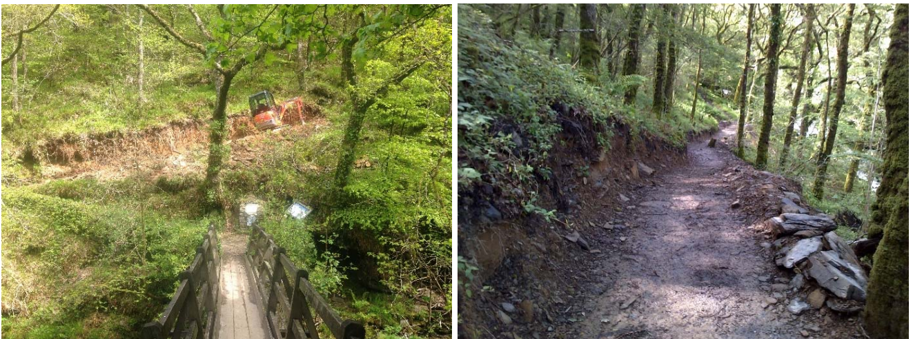
Works to replace footpath in National Trust's Wilsham Woods, Rockford
