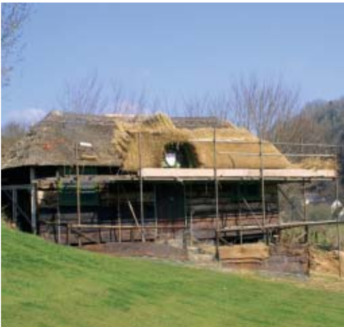
Thatching Bridgetown Cricket Pavilion (photo Heather Lowther)
