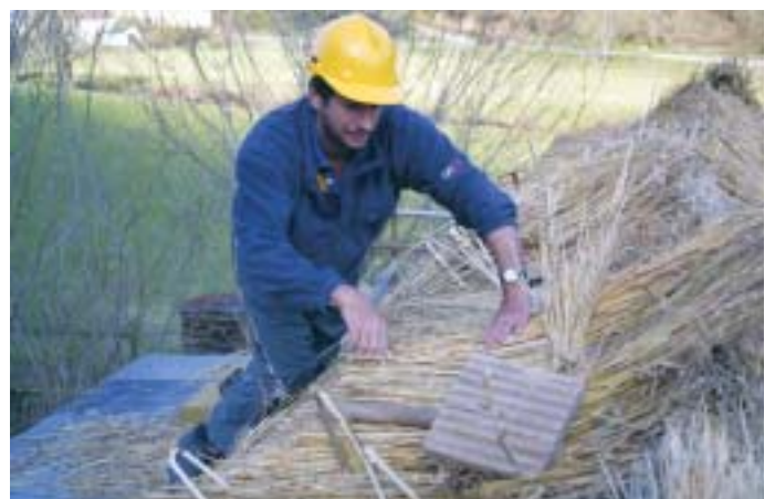
Combed wheat reed thatch being applied (photo Heather Lowther)
