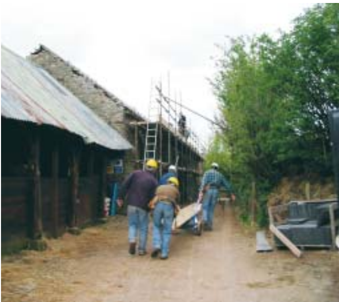
Farm building repairs carried out under DEFRA's ESA scheme (photo DEFRA)
