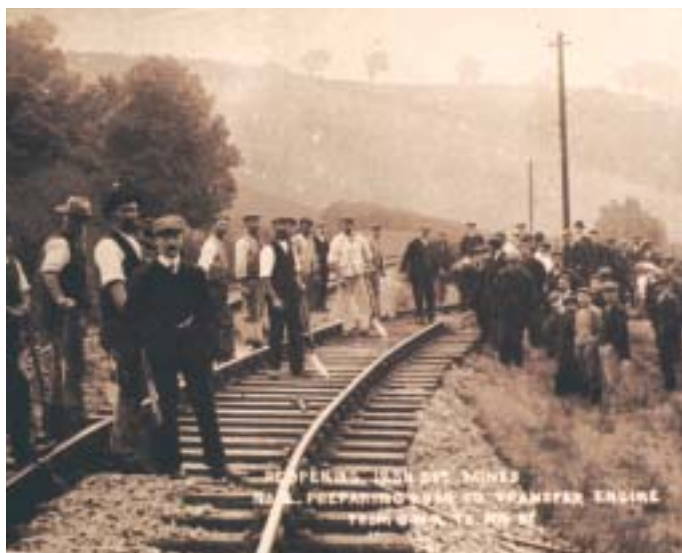
A contemporary photograph of the West Somerset Mineral Railway - one of a large collection forming a valuable, and yet largely untouched, resource.
