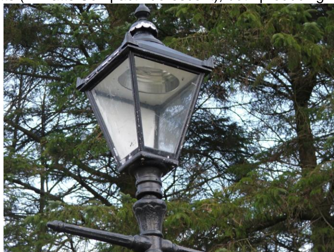
Figure 2.9 Good example of Heritage Luminaire with rear light limiter, lamp recessed in canopy hood and light distribution using pot-optic. (St Lukes Church, Simonsbath)
