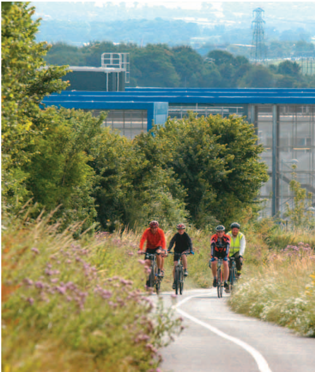
Planning obligation led to the creation of a cycle track to the new Met Office buildings in Exeter (Apex/Jim Wileman)
