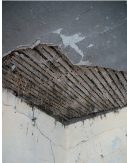
Lath and Plaster Ceiling (Photo Nicholas Dawson July 2011)
