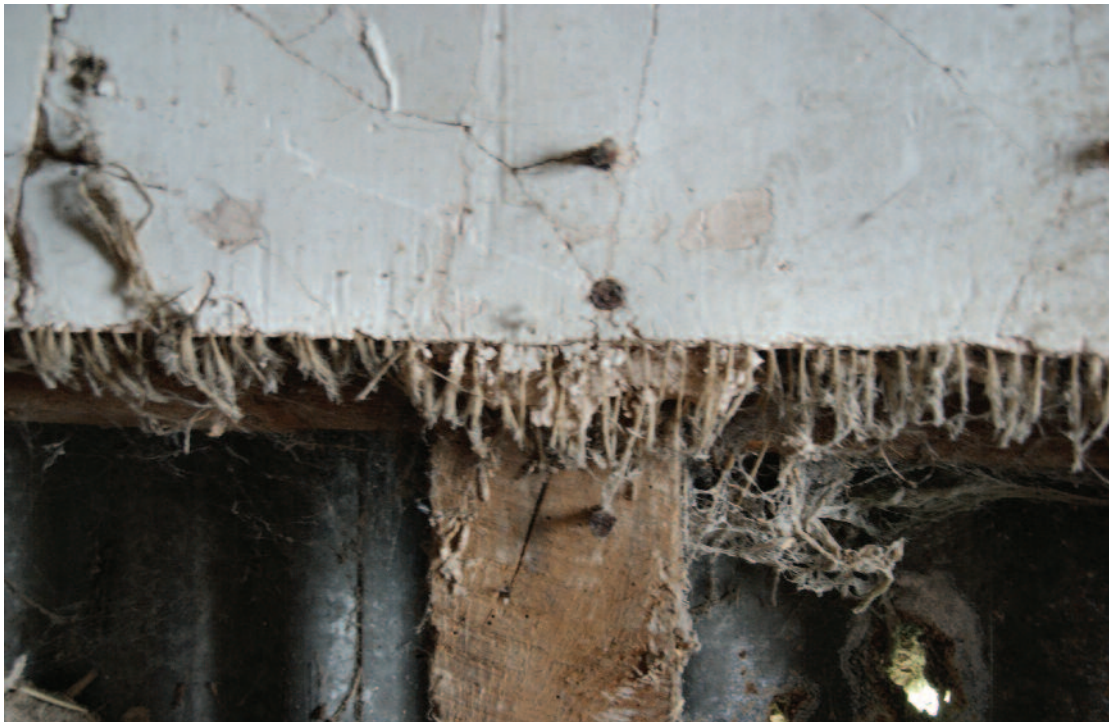
Section of plaster on hessian panelling (Photo Nicholas Dawson July 2011)
