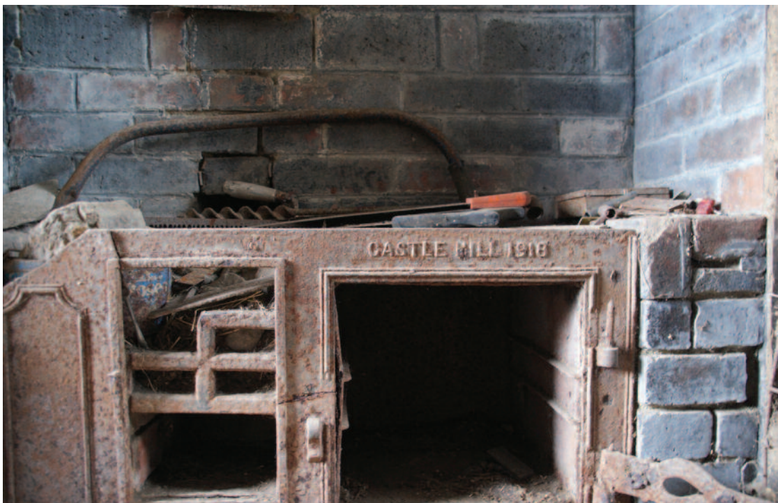
Iron range with 'Castle Hill 1918' moulded onto front, located Room 3 east wall (Photo Nicholas Dawson July 2011)
