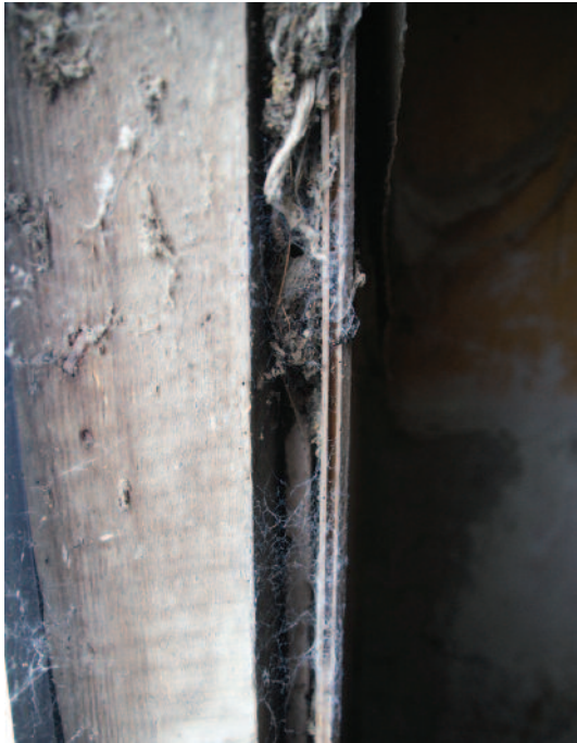
Interior wall cladding wooden panels over plaster panelling found in Rooms 1, 3 and 4 (Photo Nicholas Dawson July 2011)
