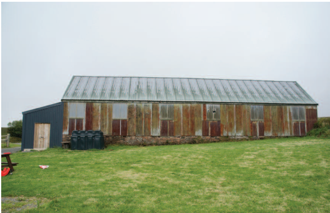
South side of the Blackpits WWI building (Photo Nicholas Dawson July 2011)
