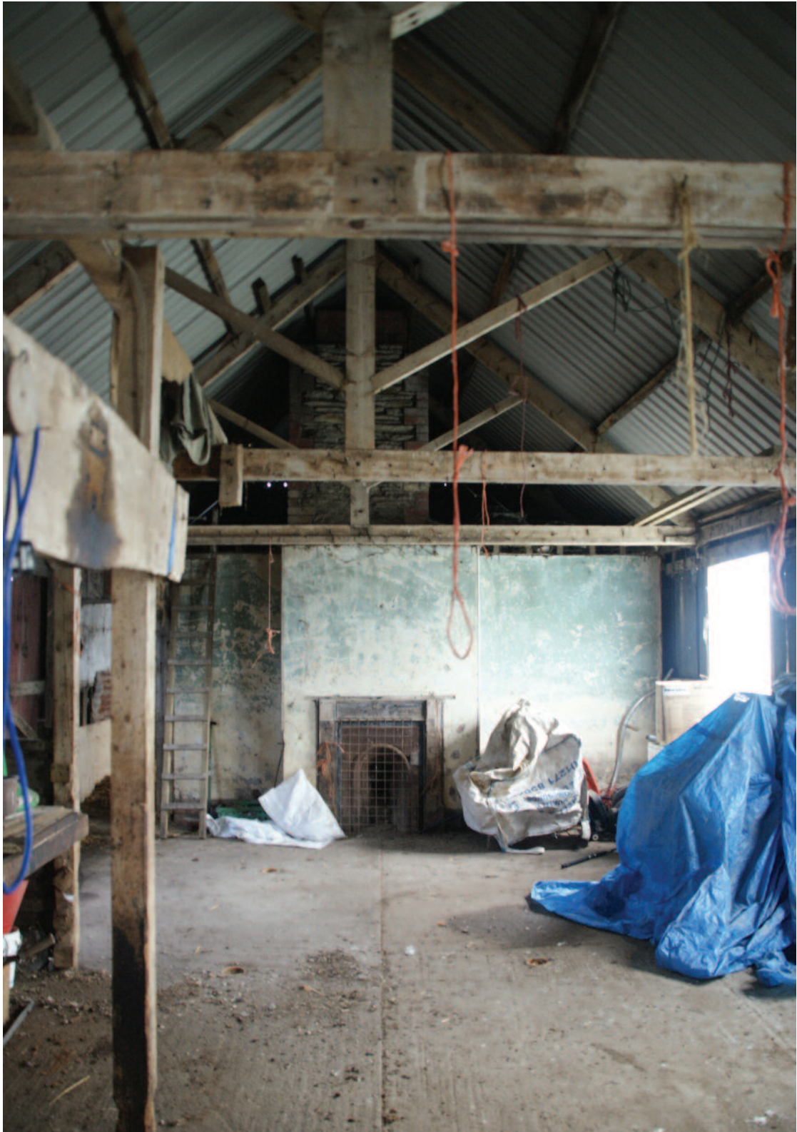
Interior of Room 2 showing the roof trusses (Photo Nicholas Dawson July 2011)
