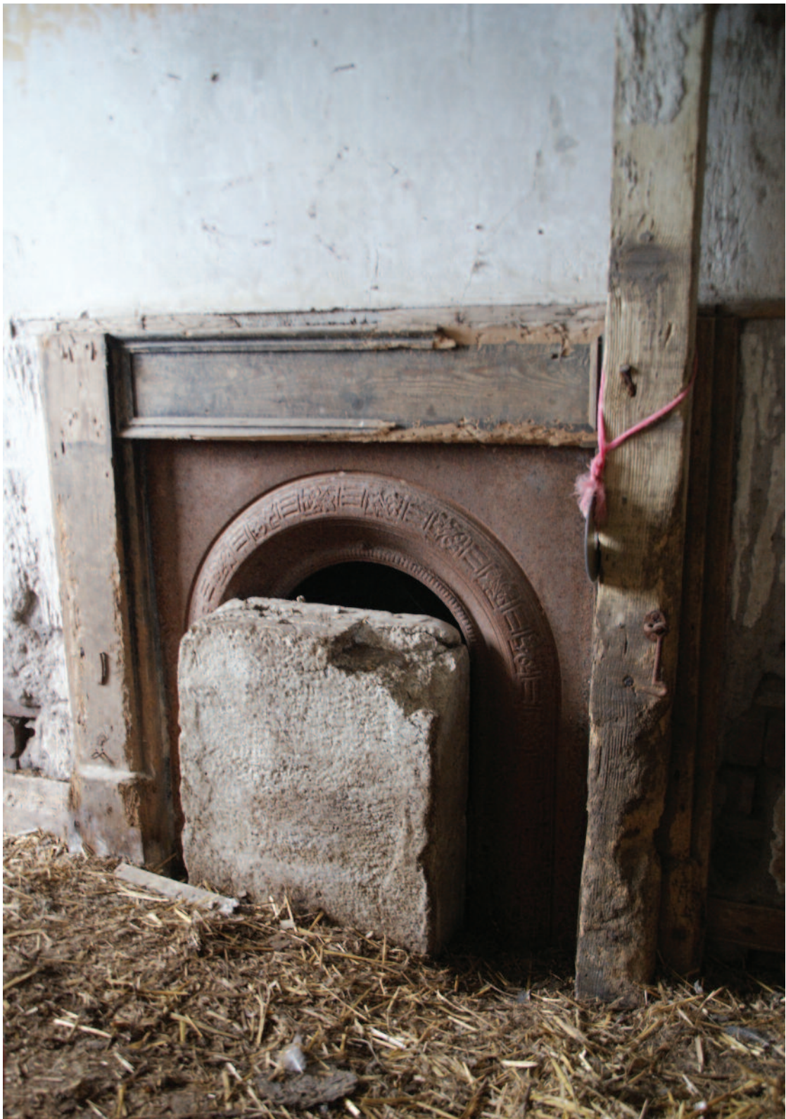
Cast iron fireplace located in Room 1, western wall (Photo Nicholas Dawson July 2011)
