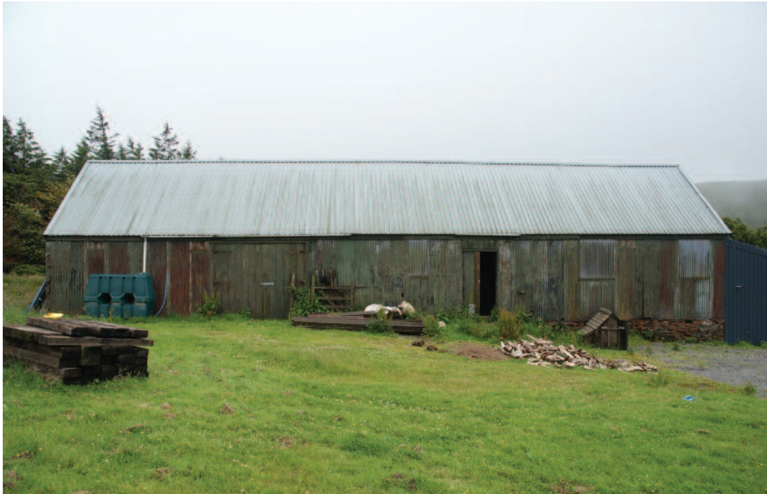
North side of the Blackpits WWI building (Photo Nicholas Dawson July 2011)
