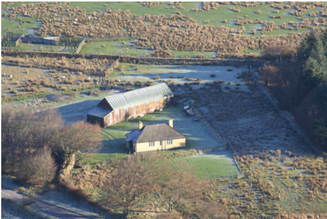
Blackpits bungalow, the WWI ex-military building and shelter belt (Photo Rob Wilson-North November 2006)
