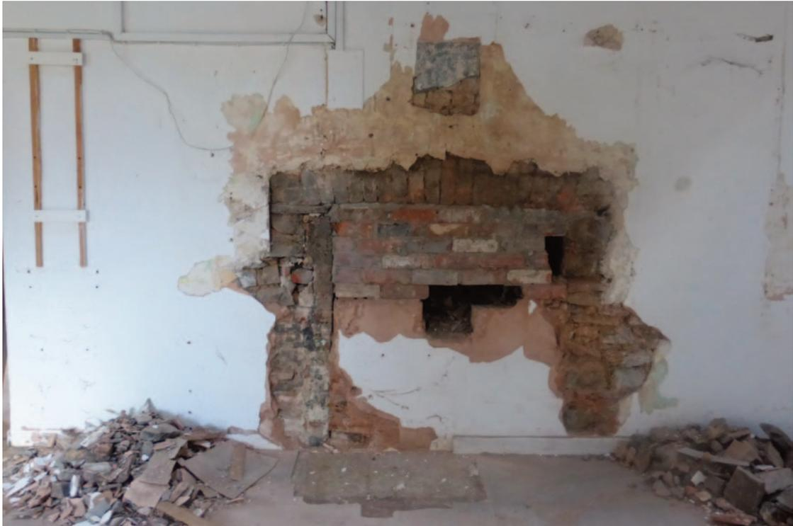
**Plate 14** The exposed outline of the original fireplace with a low brick lintel arch after further opening up. Note the strip of brick infill on the left jamb showing narrowing, the partially exposed stone floor or hearth and the slate panel 0.30m x 0.30m centrally placed above the fireplace.
