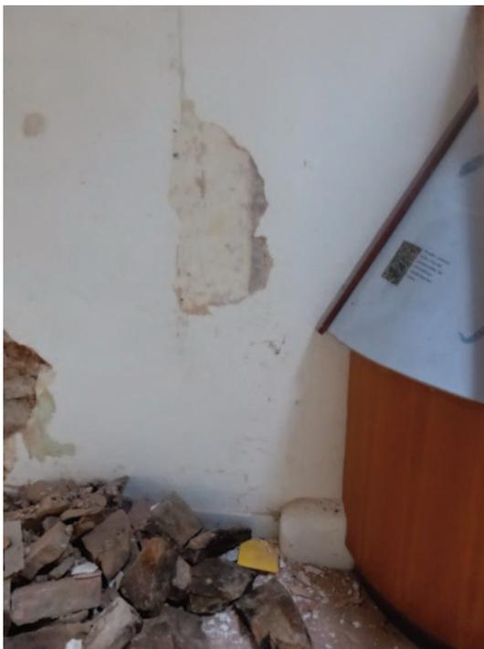
**Plate 15** The position of the north partition wall is revealed beneath the modern plaster skim, note the position in relation to the floor plinth.
