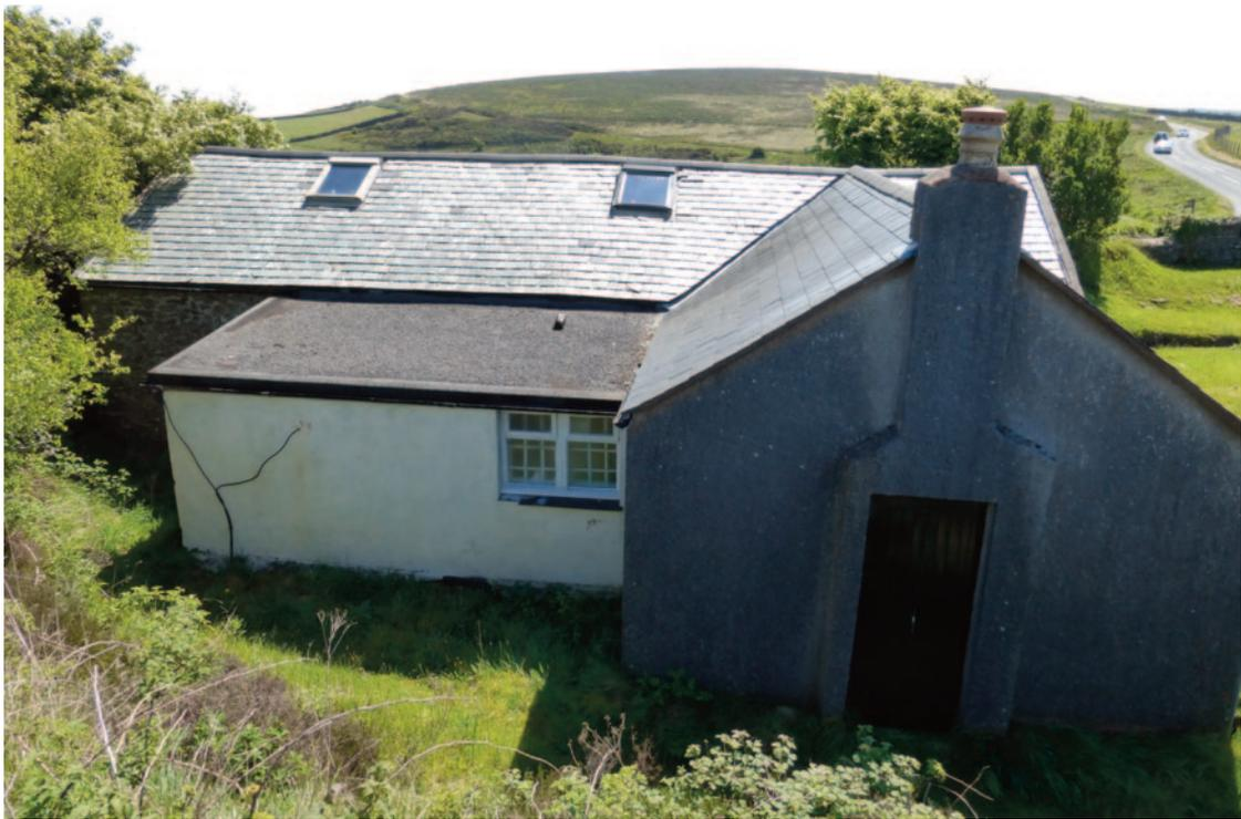
**Plate 3** The rear of the building showing the two 20th century extensions, the roof lights and the door inserted through the chimney stack in 1978.
