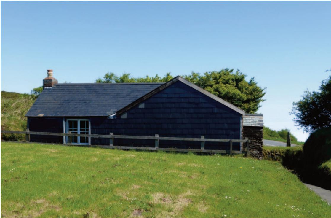
**Plate 1** The slate hanging on the southern elevation
