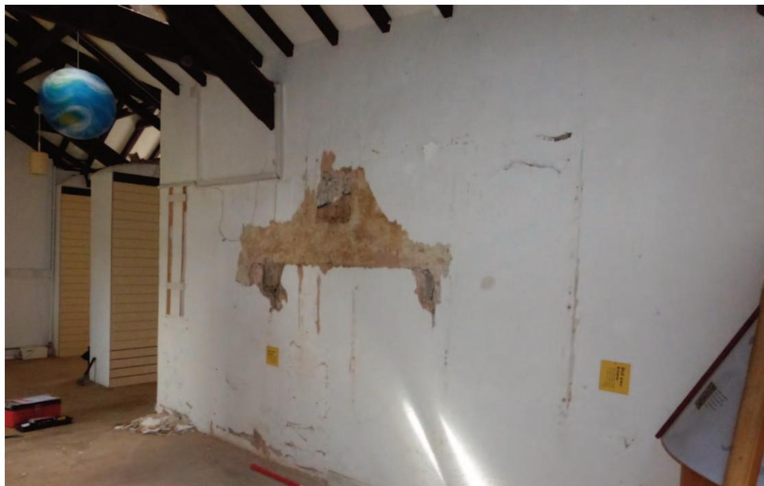
**Plate 13** The exposed outline of the fireplace in relation to the rear wall of the main range after the removal of a display panel and some paint /plaster skim.
