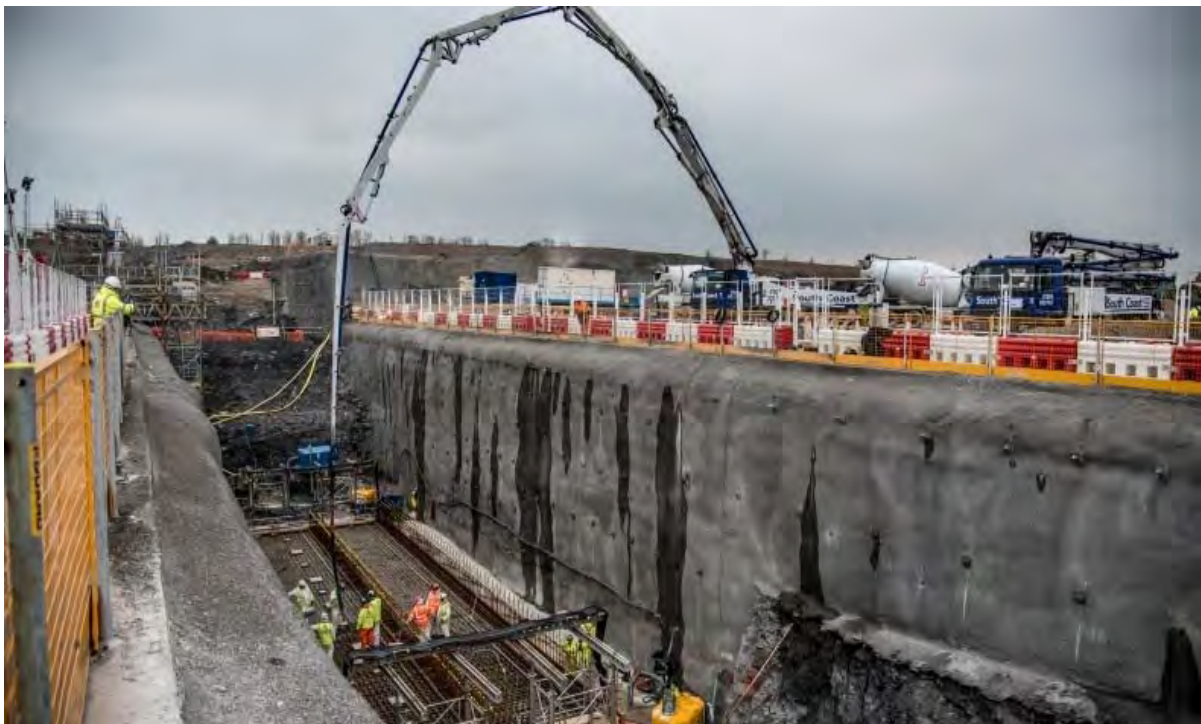
First concrete successfully poured for power station galleries © EDF Energy
