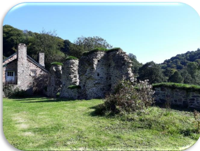
Consolidated conservation works at Barlynch Priory
