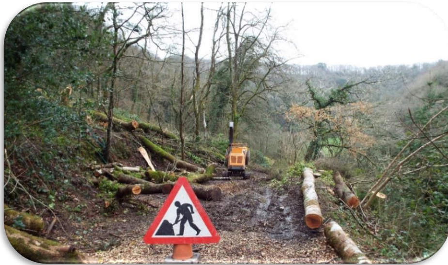
Tree felling works at Newgate Plantation due to Ash Dieback
