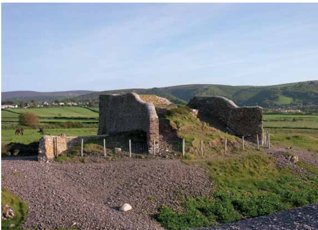
Plate 16: Post-medieval lime kiln at Bossington Beach (©ENPA 2012, G. Lawrence)
