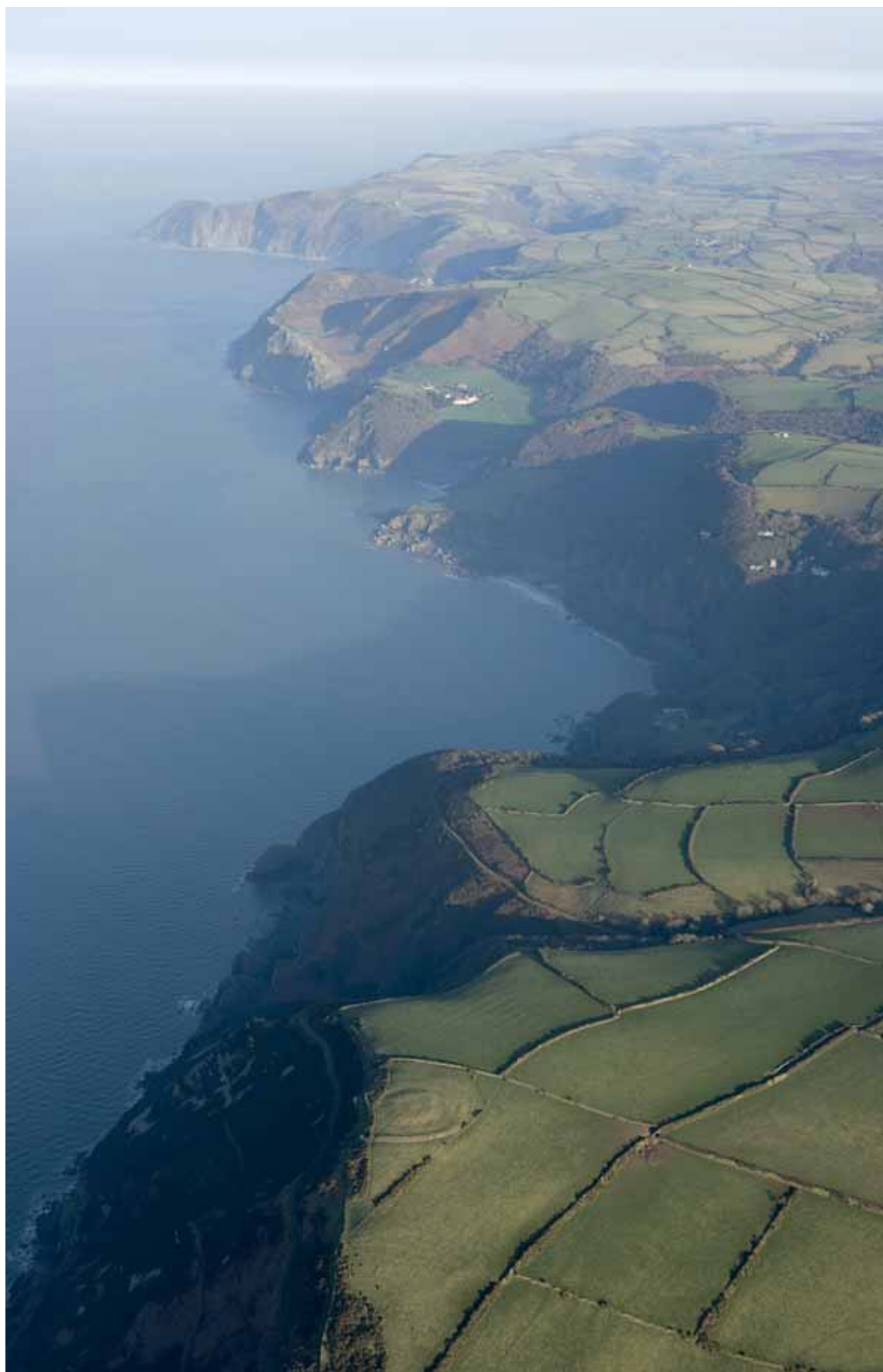
Plate 12: View along the coastline towards Foreland Point, with the earthworks of Martinhoe Roman Fortlet in the foreground (©Historic England Archive 2008, 24932_004, D. Grady)
