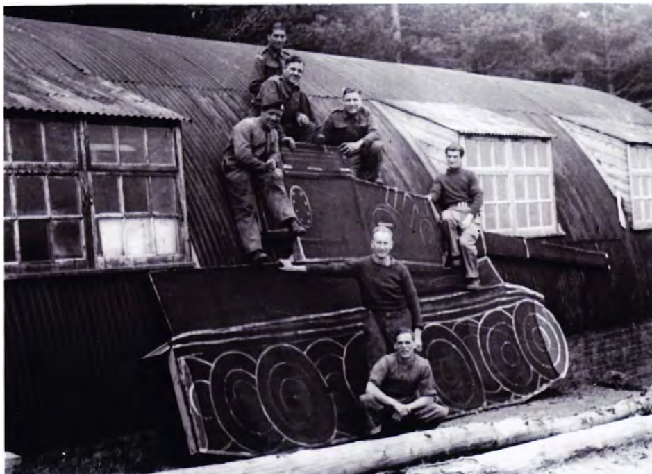
A cardboard dummy tank which ran along a light railway track. Photograph courtesy of Justin Blundell
