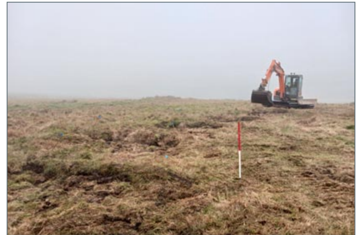
Peatland restoration work near Challacombe (c) SWPP
