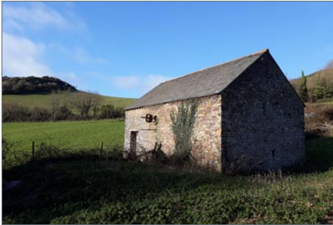
Historic farm buildings often have high landscape value, but are increasingly vulnerable
