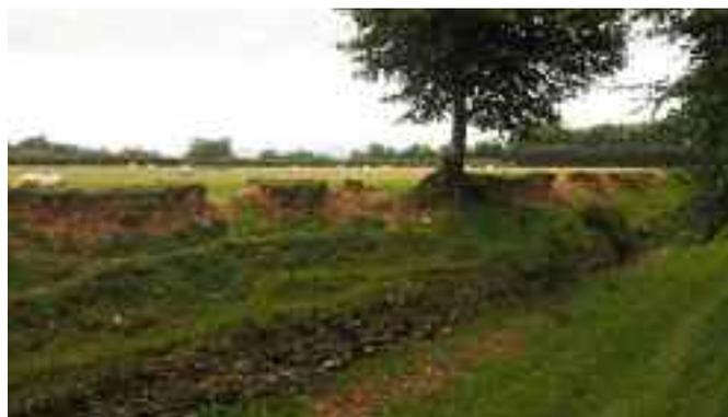
Degradation of earth bank as trees die, and tree roots are no longer able to hold the bank together
