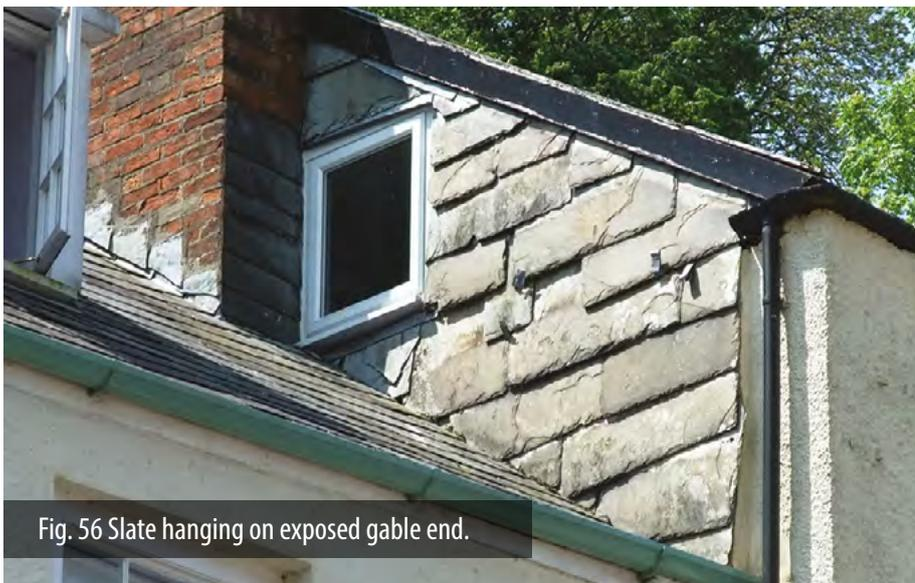
Fig. 56 Slate hanging on exposed gable end.
