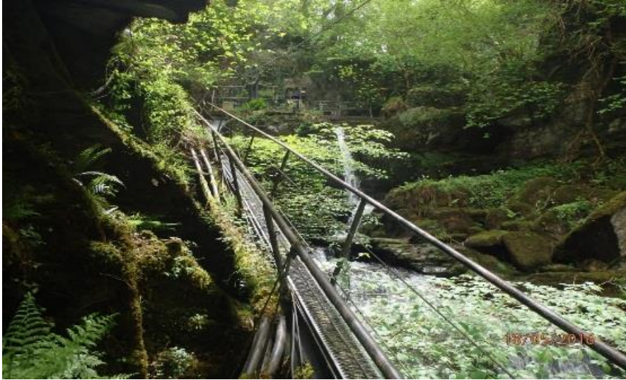
Hydroelectric facility at Glen Lyn Gorge
